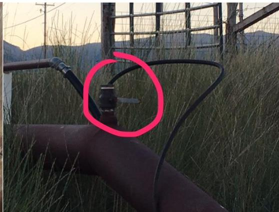
6. Remove the air lock plug from the pump until water flows out.
